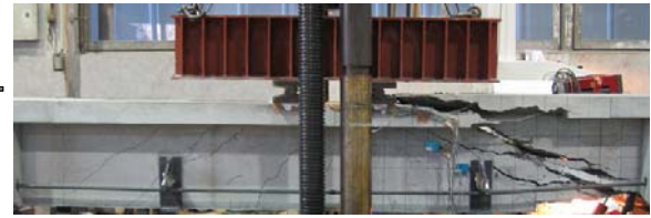
(a) Crack Patterns for ns7 (Overall beam)
