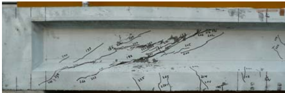
Fig. 7 Failure mode of fiber reinforced beam (PC-2.0)
