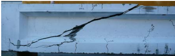
Fig. 6 Failure mode of control beam
