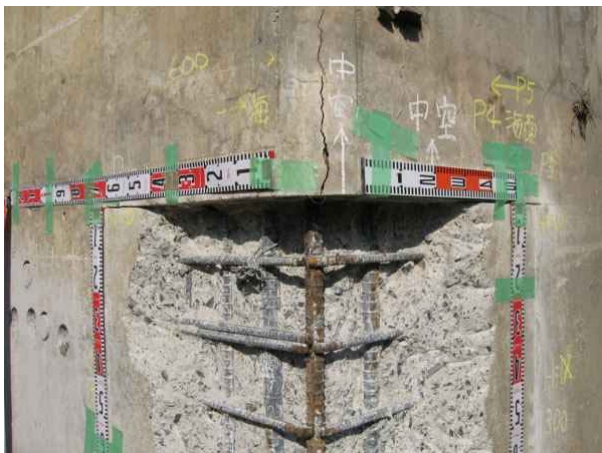
(c) 橋脚・柱 (I橋)
