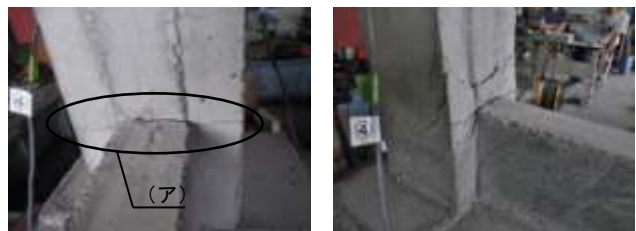
(a) R=1/100rad (b) R=1/30rad 写真-1 斜めひび割れ (F21h-30S 11 )
