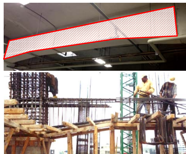
Fig. 1 RC buildings with haunched beams
