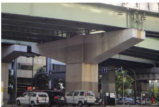
Fig. 1 Tapered RC beam in the pier structure
