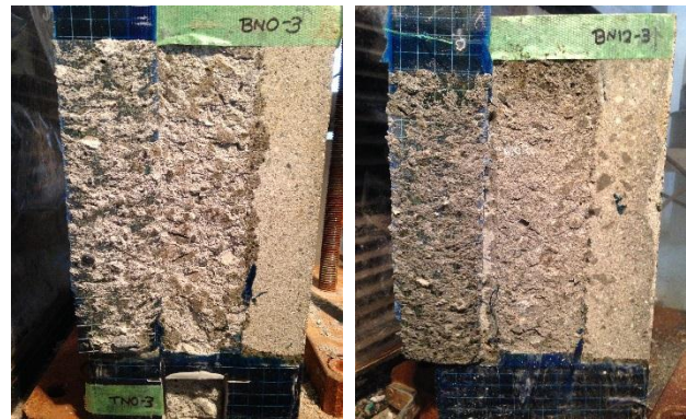
0 month 12 months Fig. 12 Concrete failure before and after the exposure (Specimen BN type)
