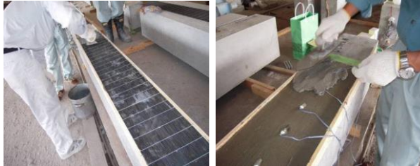
Photo.2 Attaching process of CFRP strand sheet and covering by PCM
