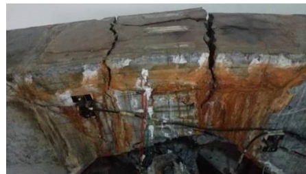
(b) Specimen of corrosion without cracks (F1)
