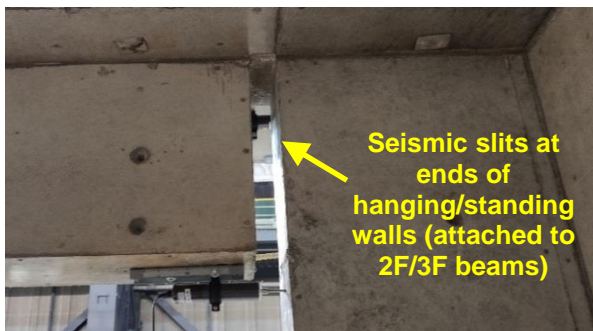
Fig.2 Detailing at hanging/standing walls ends, (a) 50 mm gap at ends of hanging/standing walls attached to 2F/3F beams, and (b) concrete filled gap on roof level beams (wall longitudinal reinforcing terminated)
