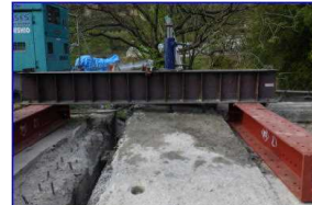
(1) RC床版撤去
