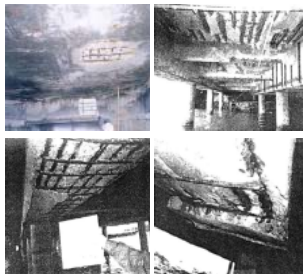
Photo 4 Deterioration Conditions
