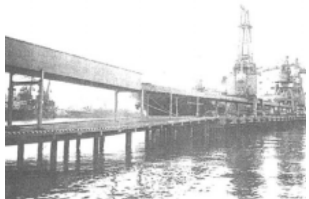
Photo 3 Panoramic view of structure
