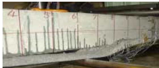
(a) Failure mode C
