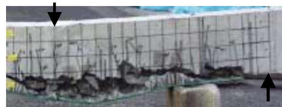
(b) Failure mode D
