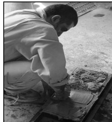
Photo 7 Casting and compaction of adobe
