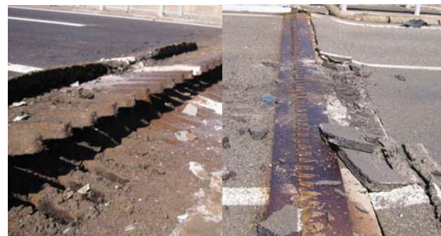
(a) P3 橋脚側 (b) A1 橋台側
