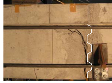
Fig. 14 Failure of shear key in SJ10-03.
