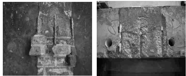
Fig.11 Anchor pullout of shear key anchors
