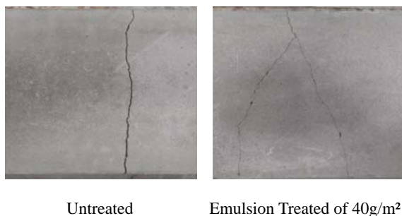
Photo 3 Cracking Tendency of Bamboo-Reinforced Cement Mortars with S50-9.
