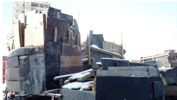
Photo 5 Large volume of waste timber at a construction site
