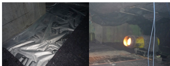
Photo 3 Curing of a concrete slab-on-grade cast in November
