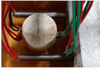
Photo 1 Sacrificial anode installed on the rebar
