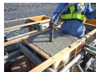
Photo 6 Situation of compaction
