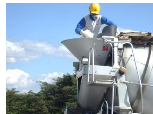
Photo 4 The throwing situation of the micro spheres to a blender
