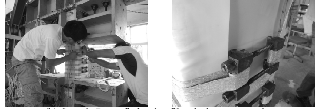
(b) Step 2: Retrofitting by fiber belts prestressing
