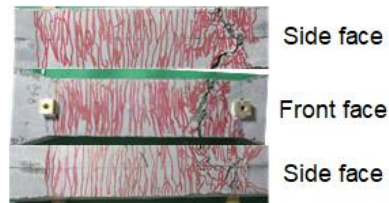
Fig.4 Cracks found in S1.0H2.0 after tension test
